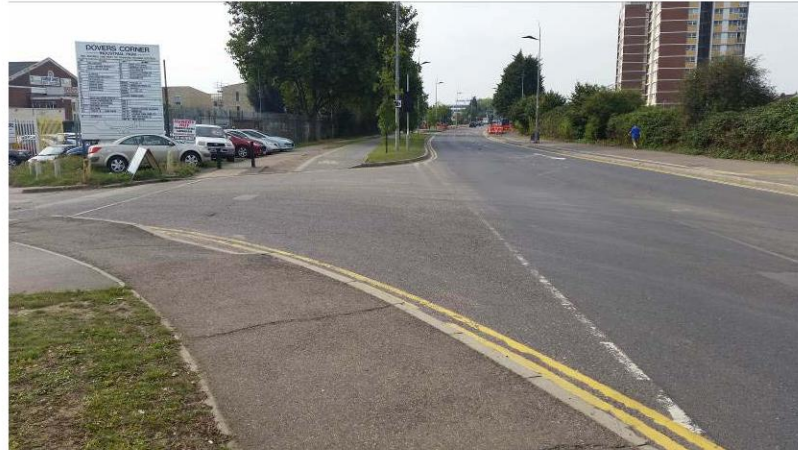
Plate 4: Primary New Road Access
