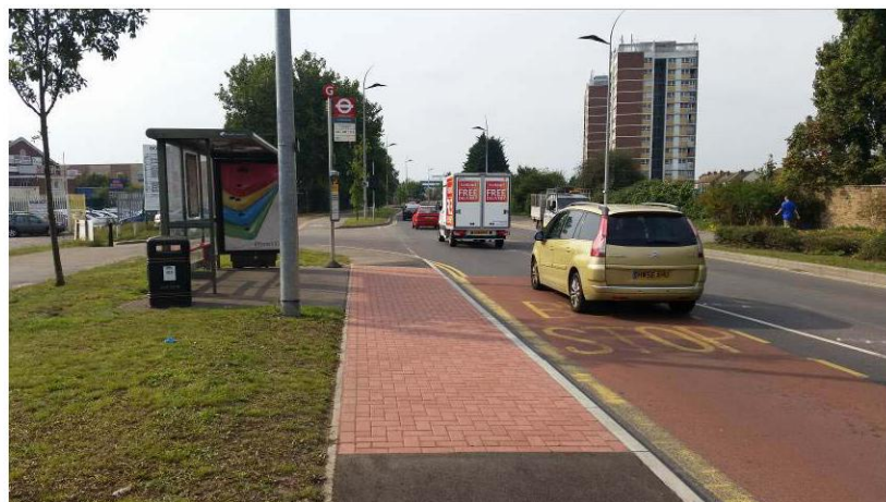
Plate 16: New Road Westbound Bus Stop
